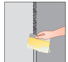
Finish the sealing with a wet spatula
