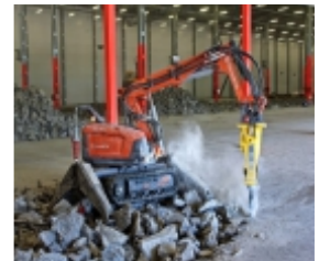
RCC Floor Demolishing
