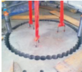
Stitch Core Drilling
