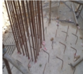
Re-Bar Grouting
