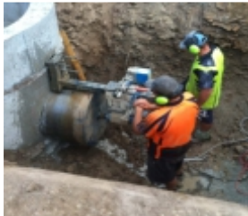
CoreDrilling
