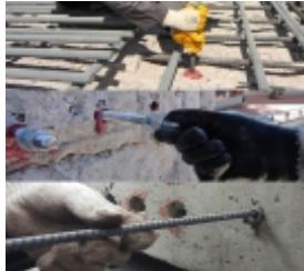
Stud Anchor Bolt Fixing
