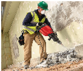
Concrete Wall Demolishing
