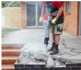
Concrete Floor Demolishing
