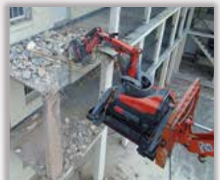
Demolishing Support
